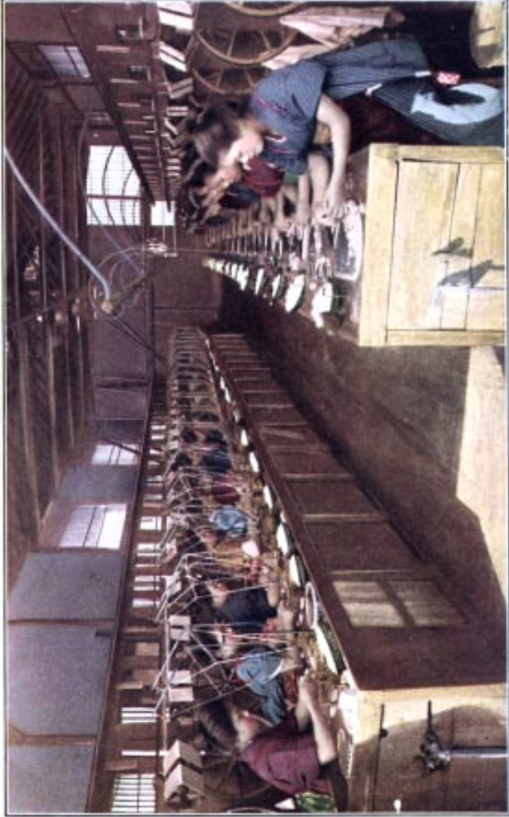
A FILATURE—REELING THE SILK FROM CORTICELLI COCOONS BY POWER MACHINERY.
