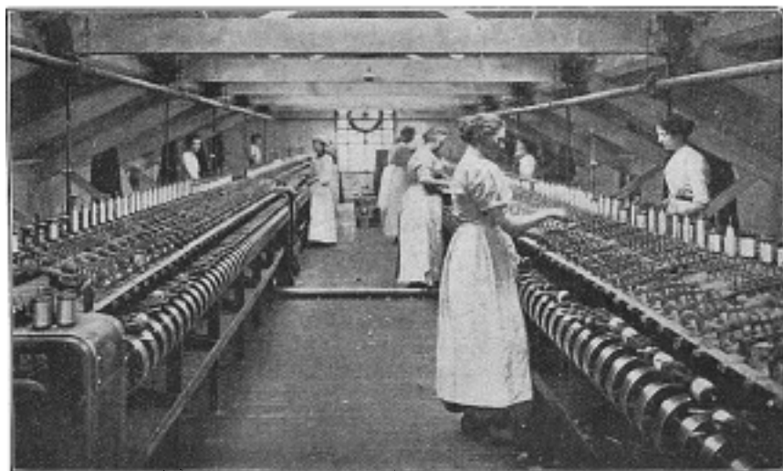
GASSING AND CLEARING SPUN SILK YARN
