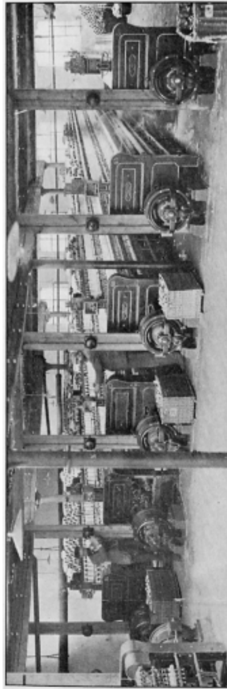
FIG. 4.—DIRECT DRIVEN RING SPINNING FRAMES, SINGLE-PHASE REPULSION MOTORS BY MESSRS. SIEMENS BROS., LTD.
